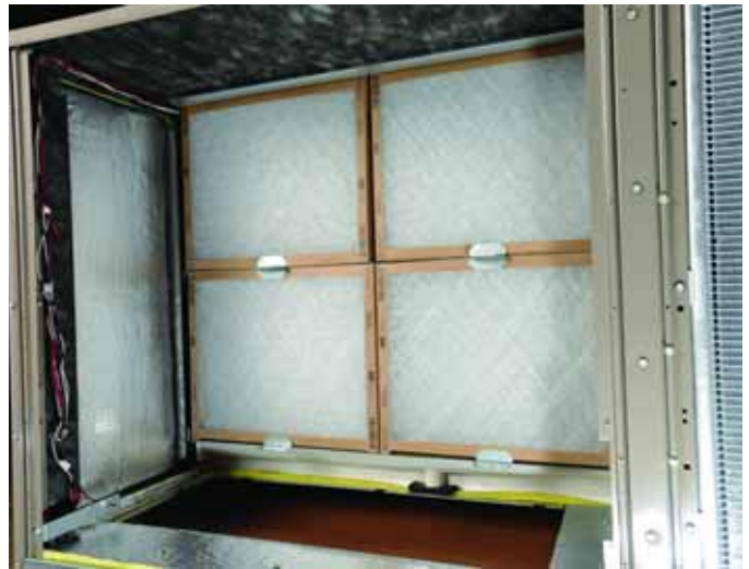
Figure 13: Bottom Return Opening For Side Duct Conversion
